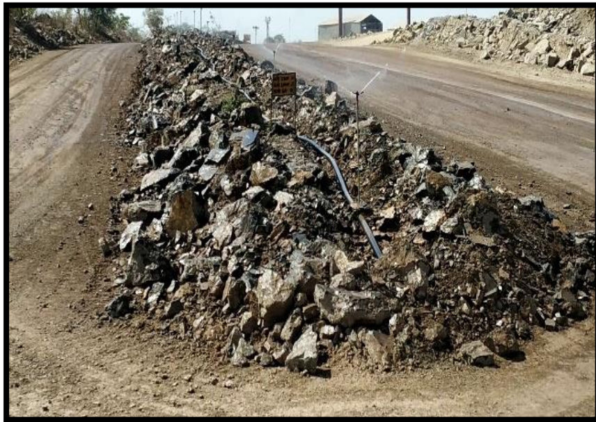
Fixed Sprinkling system
